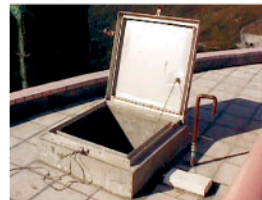
Water Tank with Raised Neck & Double-sealed Cover
