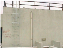
Properly Maintained Water Pipe
