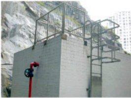
Water Tank with Proper Maintenance
