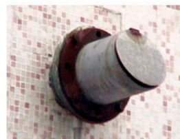
Overflow Pipe with Self-closing Lid
