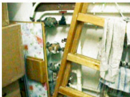
Inaccessible Water Meters
