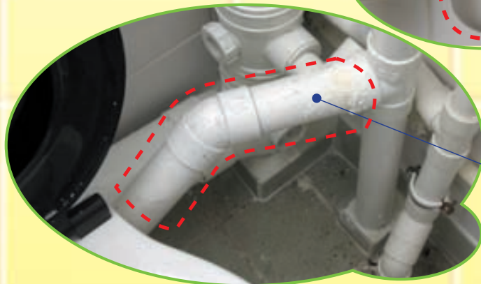
備有反虹吸氣閥的隔氣彎管 Trap with anti-syphonage air valve
