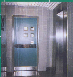
Fireman's lift lobby
