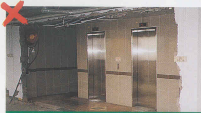
Removal of fireman's lift lobby
