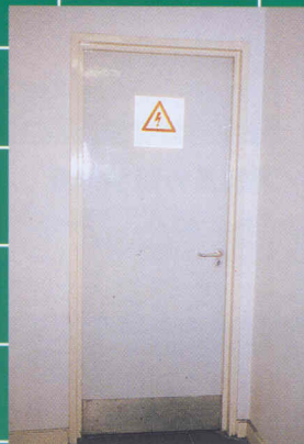
Special hazard room
