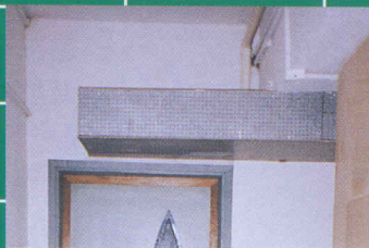
Cable and duct protection
