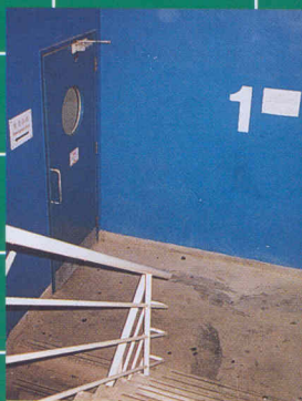
Staircase and fire door
